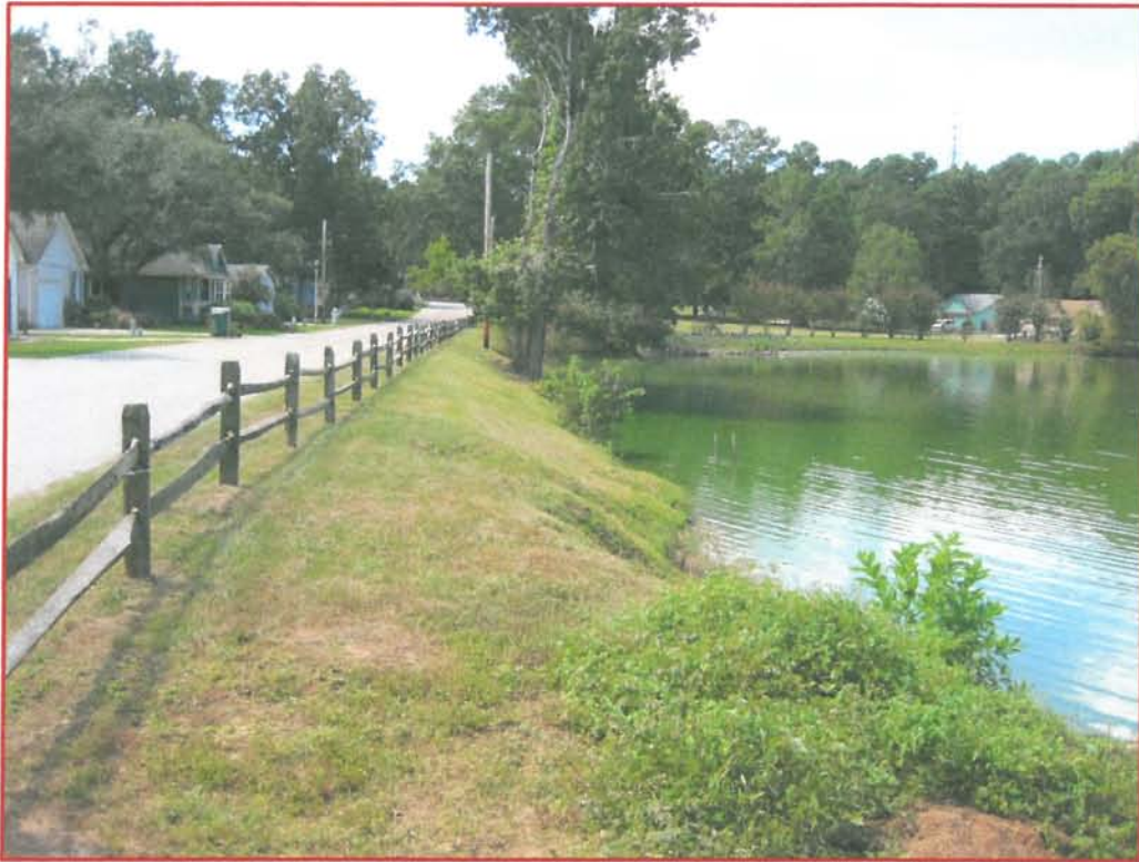
FIGURE 3C: VIEW OF SOUTHERN SLOPE OF THE EXISTING POND (FACING WEST)
