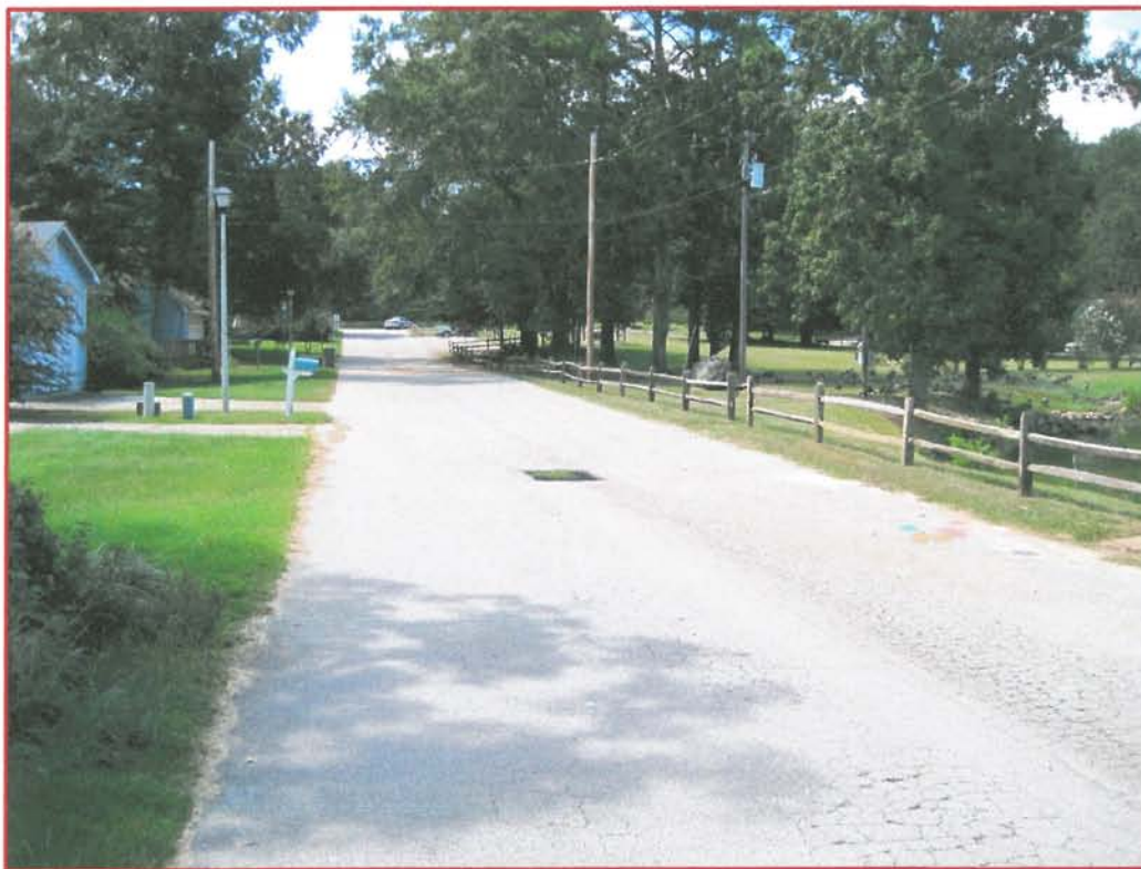
FIGURE 3B: VIEW OF DRAINAGE INLET LEADING TO THE EXISTING POND (FACING WEST)
