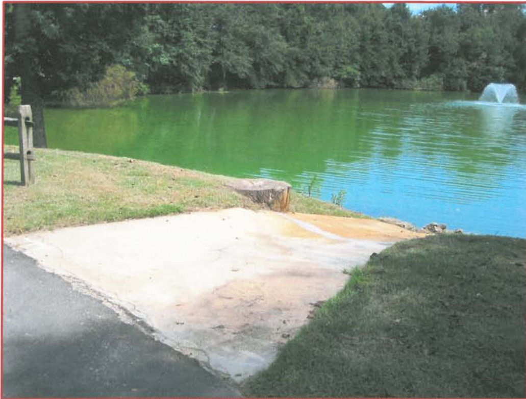
FIGURE 3D: VIEW OF CONCRETE DRAINAGE DITCH (FACING EAST)
